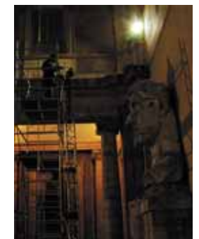
Laser scanner and structured light scanner during submillimetre-accuracy 3D documentation. (Photos & graphics: ArcTron 3D GmbH).
